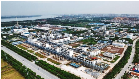
New Jingzhou site encompasses 16 buildings as well as other infrastructure, including a wastewater treatment facility
